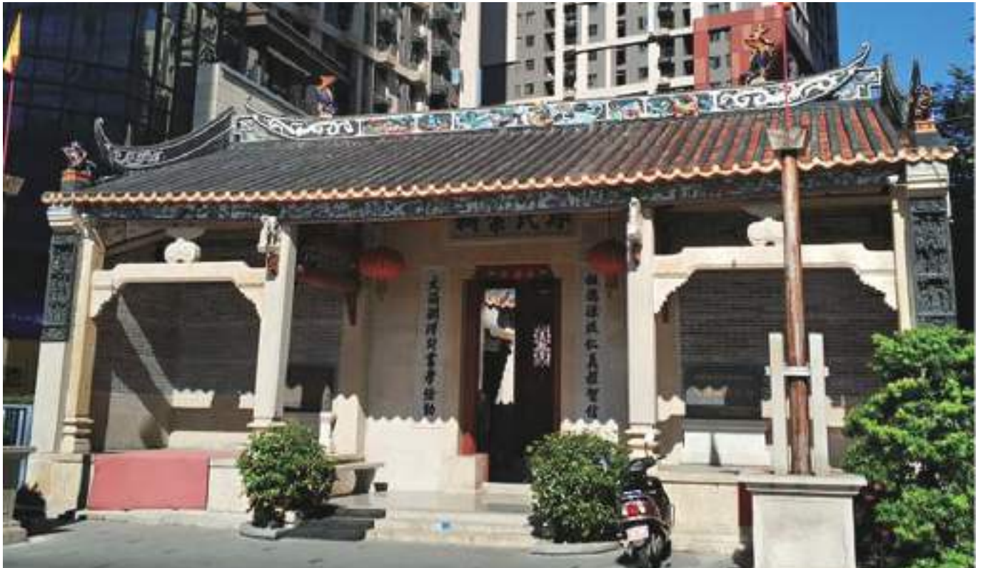
Picture of the Ancestral Hall of Family Zheng after Repair Works
