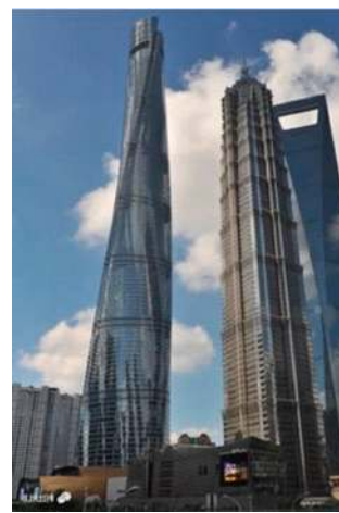
Shanghai Tower—Double glazed curtain wall system, featuring glass curtain wall units mounted on a set of gravity steel rod and steel ring beam structural system.
