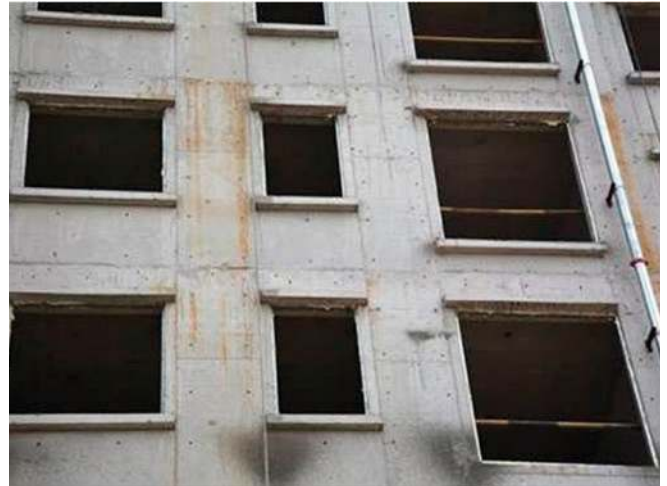
Embedded steel subframe
