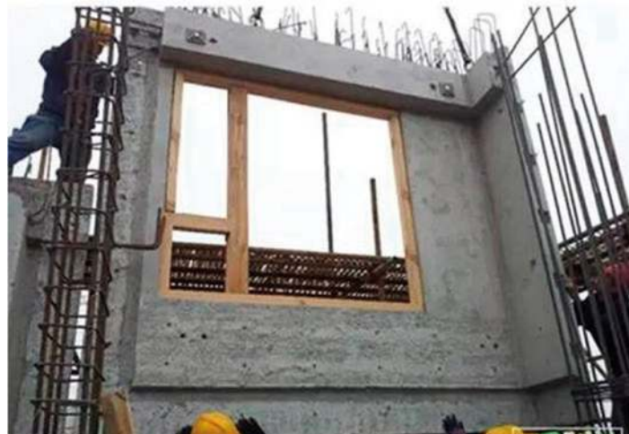
Door and window frames completely embedded
