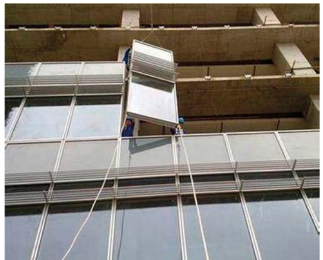
Installation of unitized curtain wall
