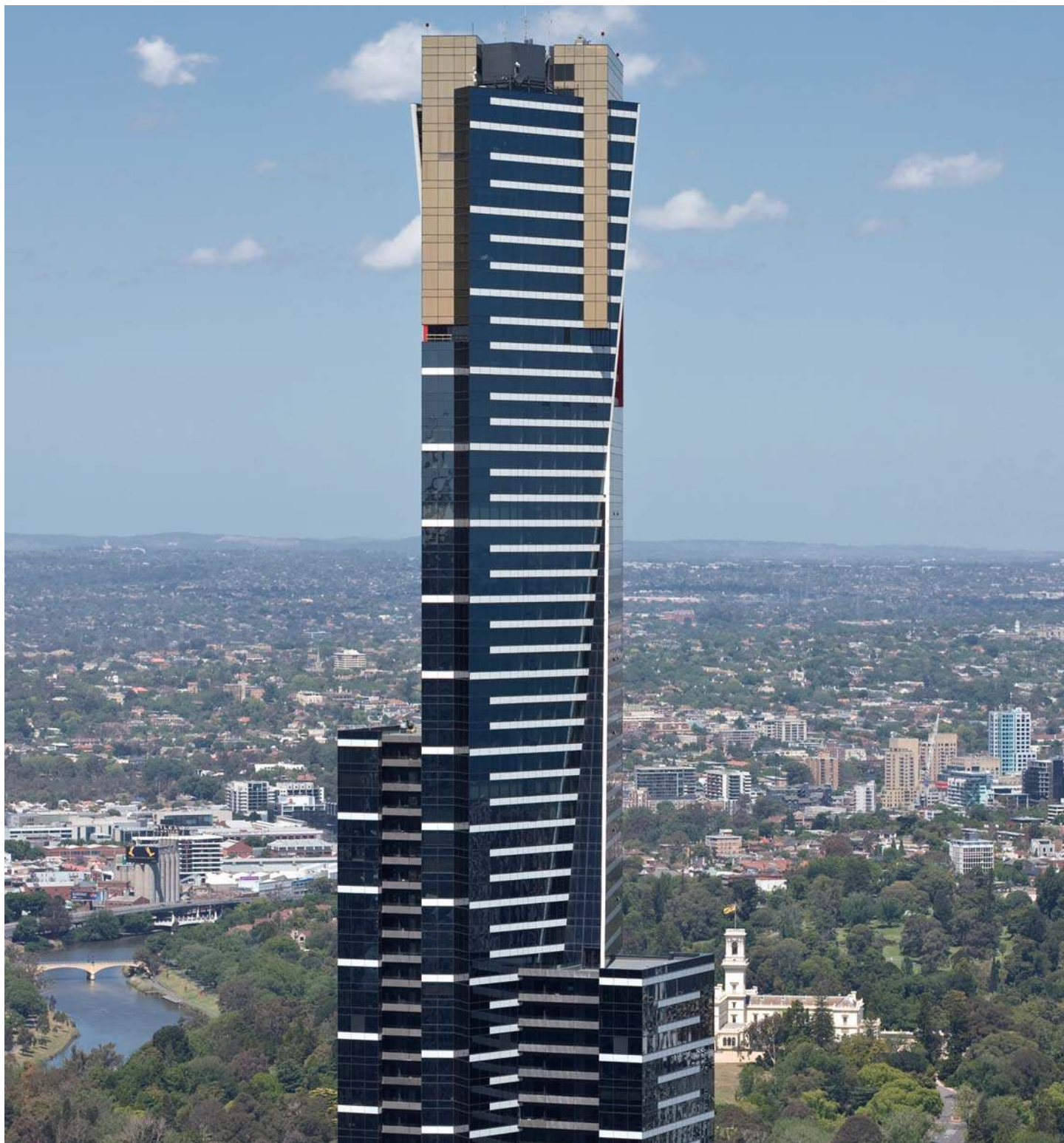
EUREKA TOWER MELBOURNE, AUSTRALIA
