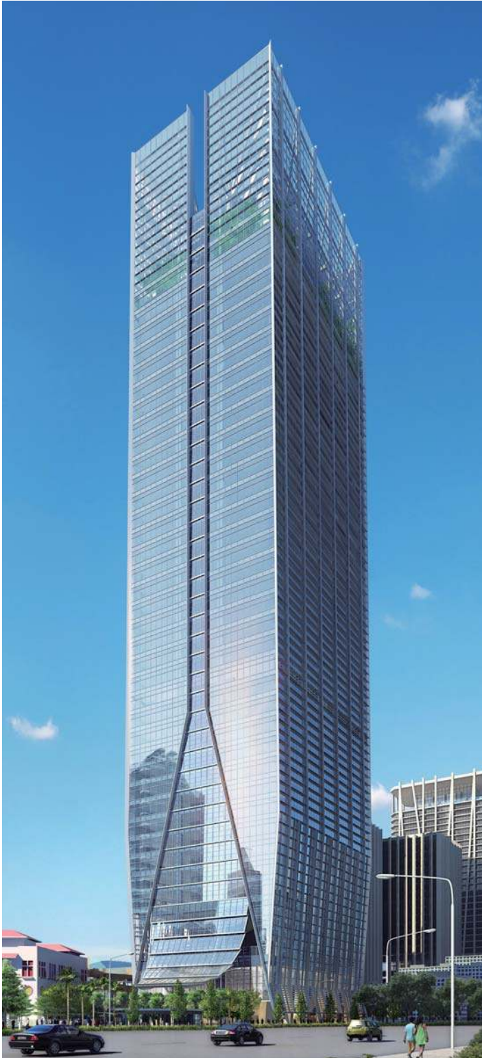
FRASERS TOWER SINGAPORE
