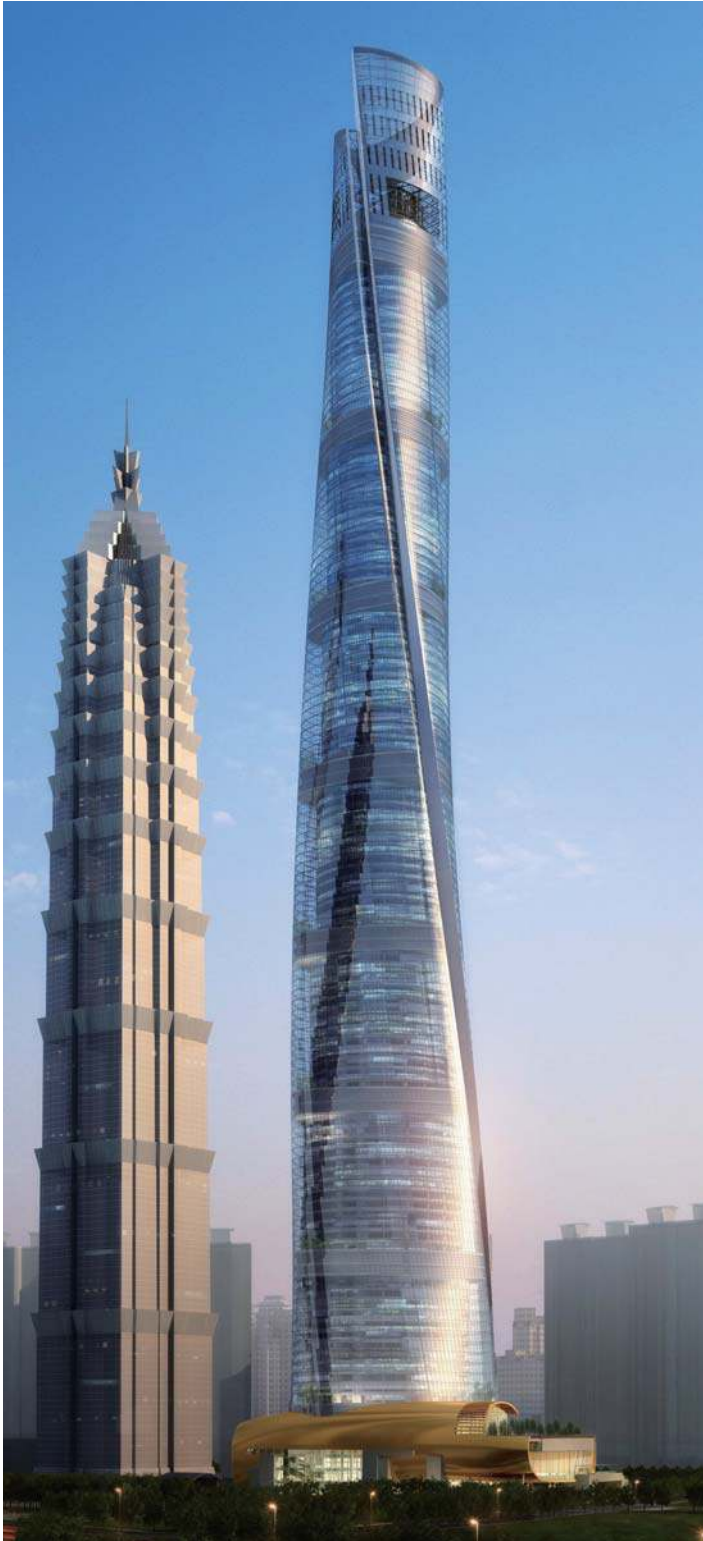
SHANGHAI TOWER SHANGHAI, CHINA
