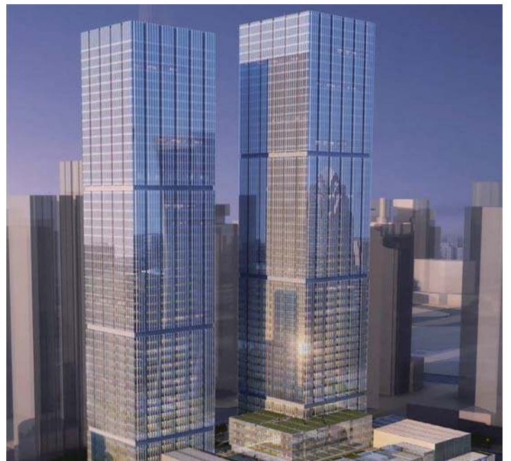
CITIC RUIBO TOWER 1 AND 2 SHANGHAI, CHINA
