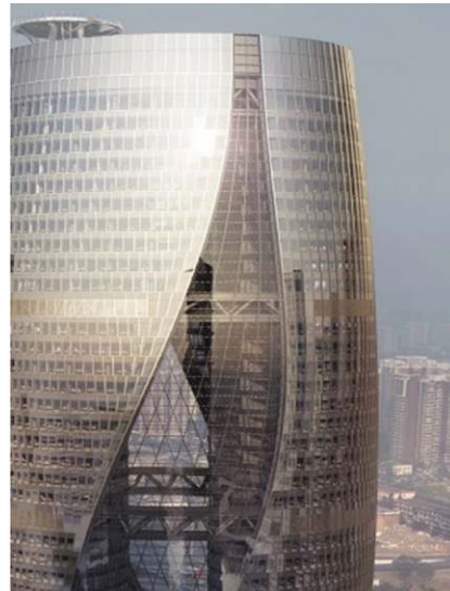
Fish scale curtain wall and point curtain wall
